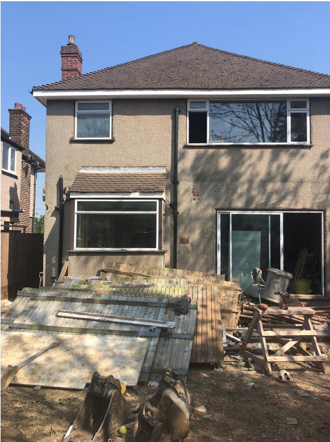
Figure 2 – Existing rear elevation of subject dwelling
