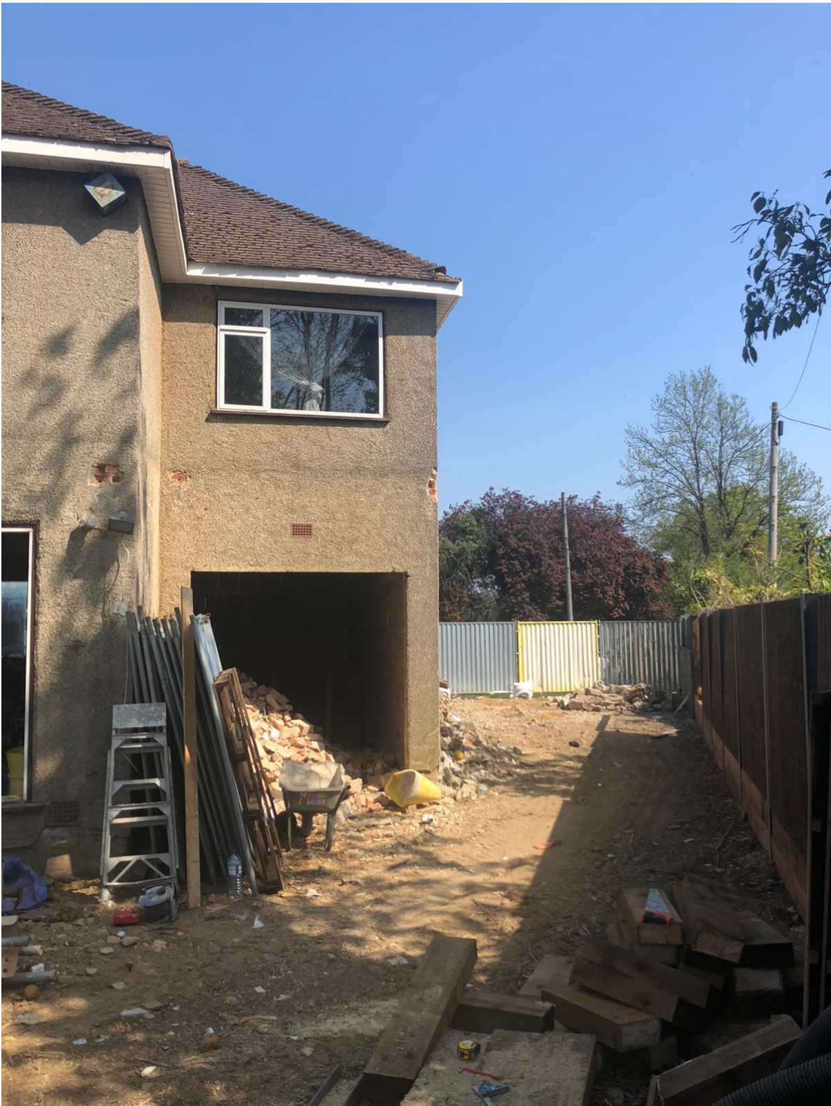
Figure 3 – Existing rear elevation of subject dwelling and existing side boundary
