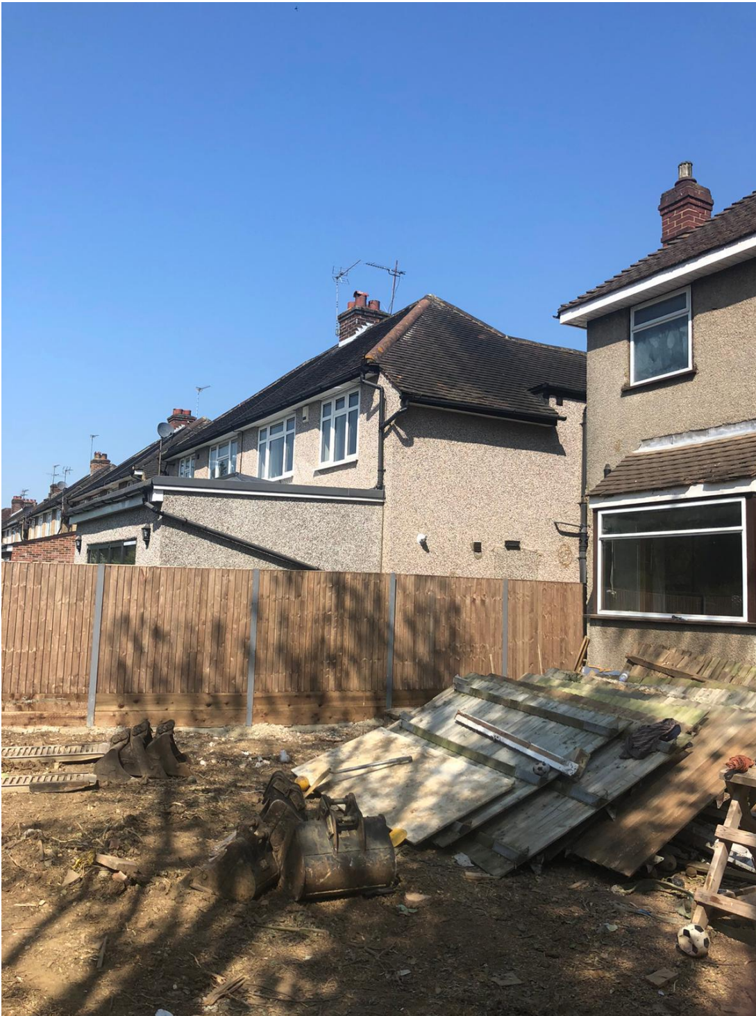
Figure 4 – Existing side elevation of neighbour at No 24 Abercorn Road
